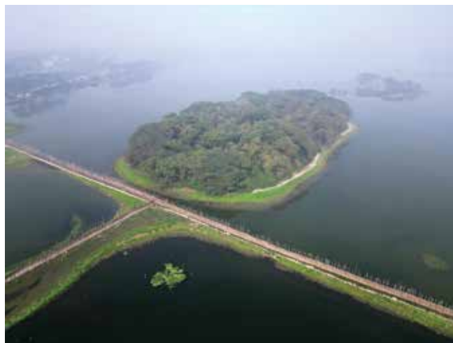
Goranchatbari Retention Pond with island
