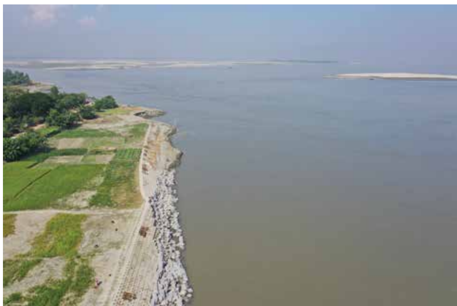
River Protection Works in the Eroded Bank of the Jamuna River near Kulkandi Union, Islampur Upazila under Jamalpur District
