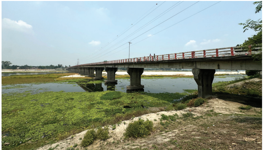
Khanshama Zia Bridge over Karatoya River, Khanshama, Dinajpur
