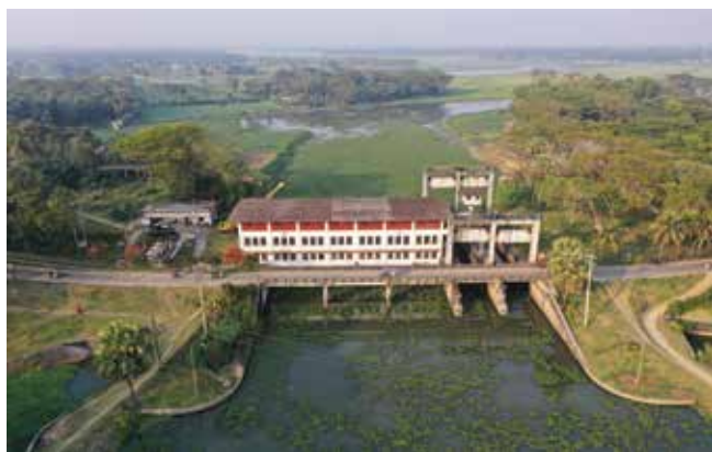
Charbagadi Pump House under Chandpur Irrigation Project
